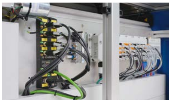
Fig. 6: The Safety Fieldbox simplifies the integration of safety switchgear into the safety circuit
